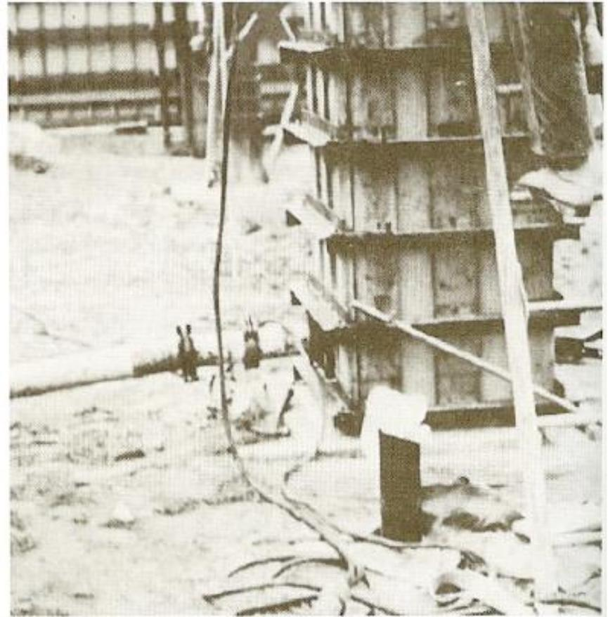
b. Pumping hose in place on fixture at bottom of form 9
