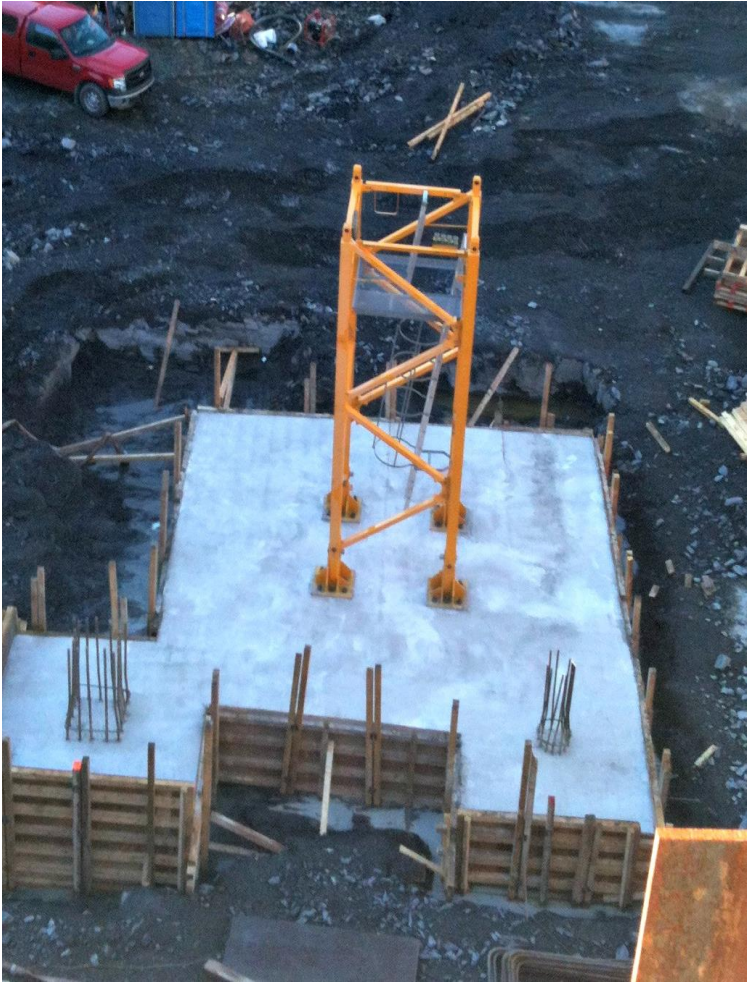
Static tower cranes
