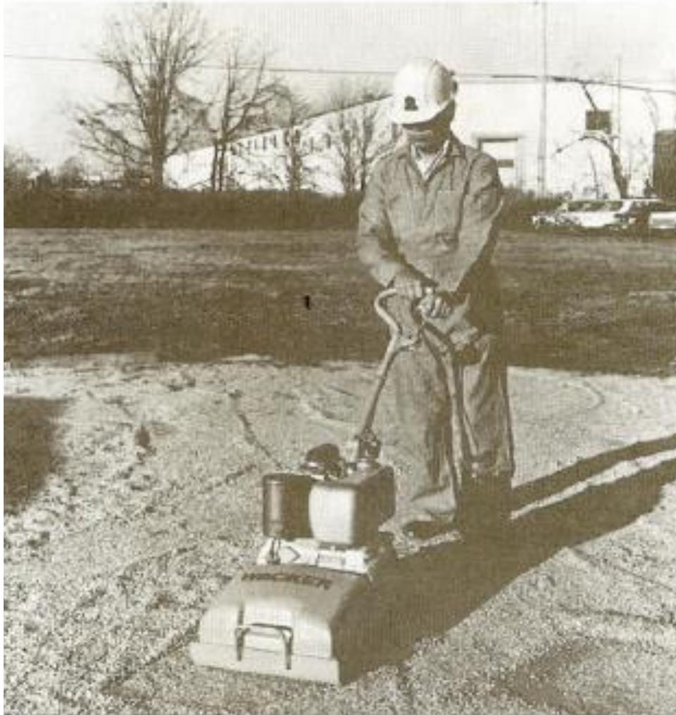
**FIGURE 5-7:** Walk-behind vibratory roller with remote control.
