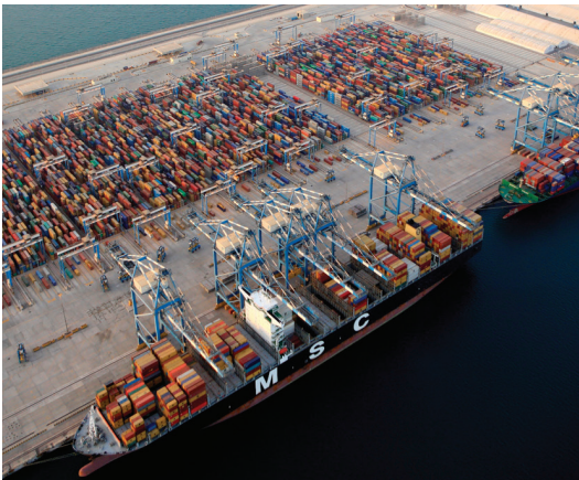
Khalifa Port, Abu Dhabi Source: Abu Dhabi Ports
