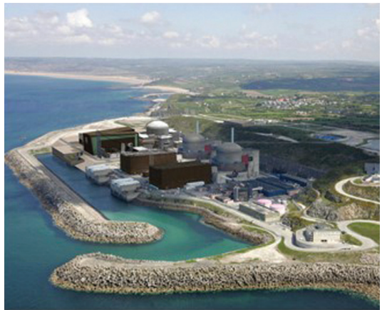
Flamanville nuclear power station Source: EDF
