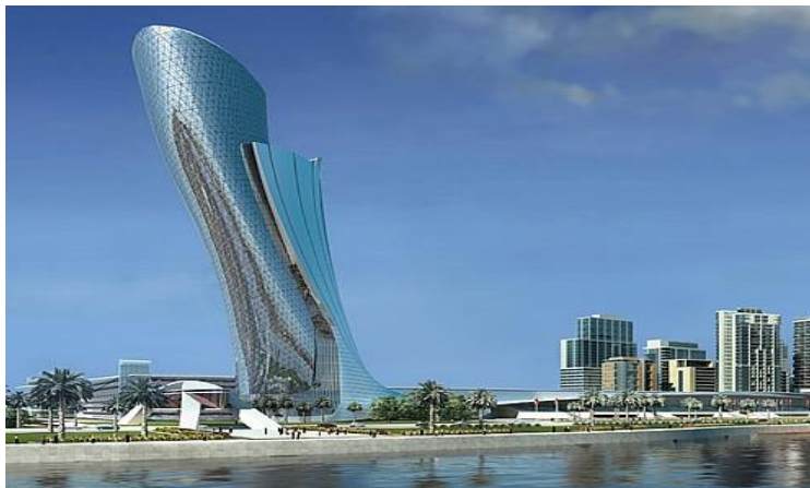
Figure 5(above), Capital Gate, Abu Dhabi, Designed by RMJM. Figure 6(right), Burj Khalifa, Dubai, Designed by Adrian smith.
