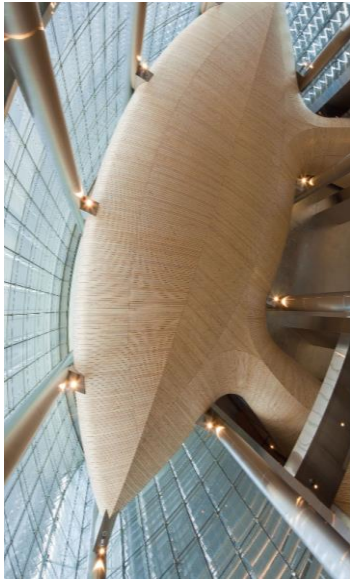
Figure 24, Burj Khalifa Foyer, Sustainable Natural Lighting through Horizontal Louvers (Courtesy of Adrian Smith +Gordon Gill).
