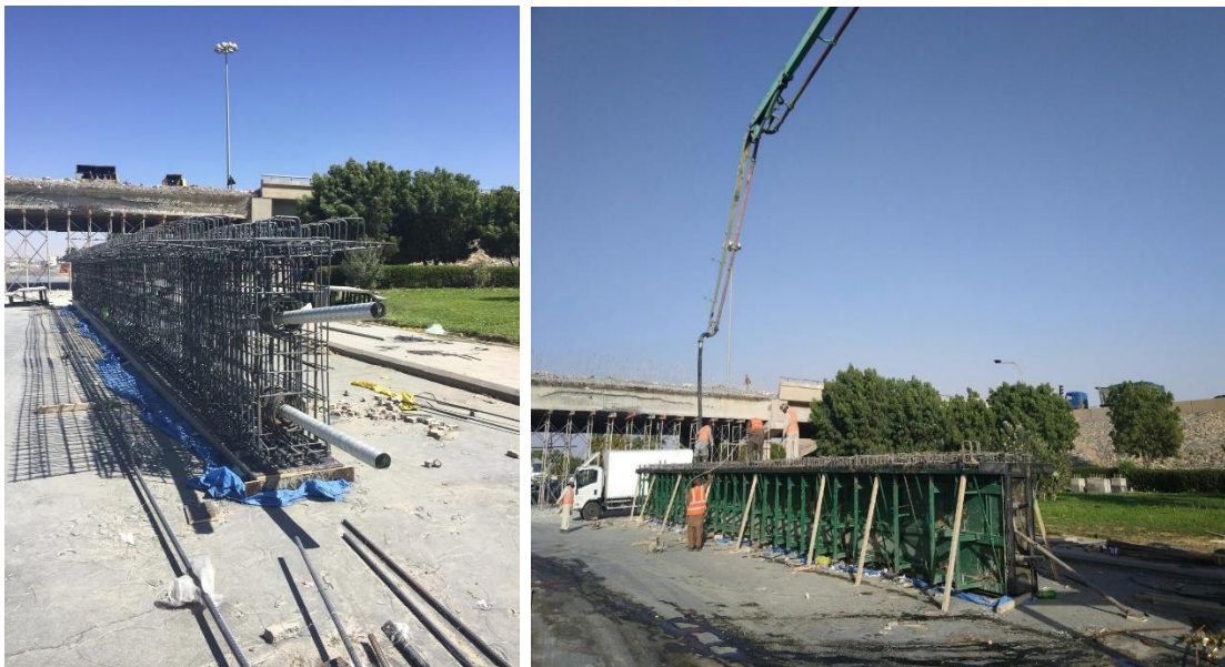
Figure 10.4: construction & casting concrete girder
