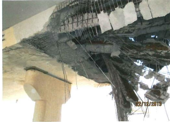
Picture of (Over Height Accidents) Picture of (Corrosion in Concrete Bridges)
