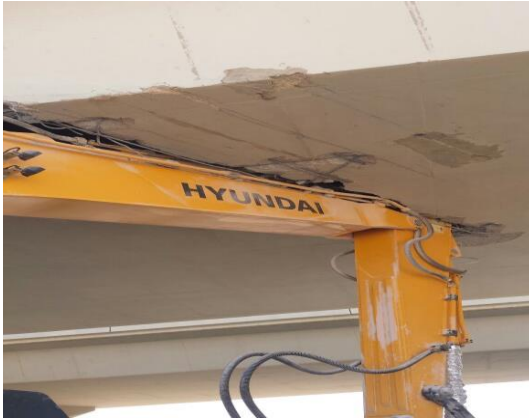
Picture of (Over Height Accidents) Picture of (Corrosion in Concrete Bridges)
