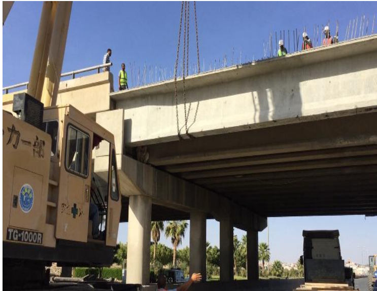
Figure 10.5: Replacement the girder
